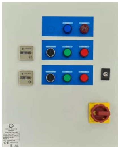
EXAMPLE TWIN PUMP PANEL
